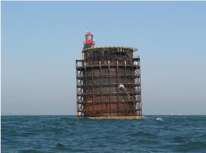
It was decided to make use of the tower. In 1920 it was towed to its new site by two paddle wheel tugs, it was to replace the Nab light vessel, by sinking it at the eastern approaches to the Solent. It was a calm day and the tower was installed with no mishaps apart from a 3degree tilt towards the northeast, it still stands at the same angle to this day.
